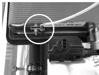
Removing the hot water return sensor
