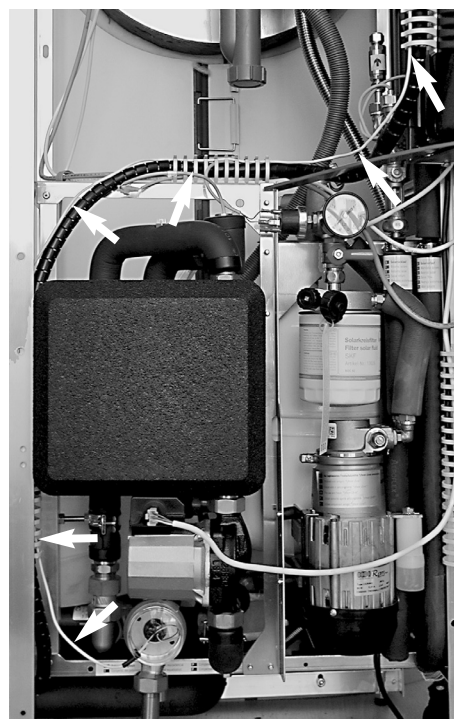
Routing the VSG-W line
