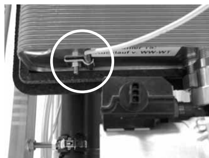
Removing the hot water return sensor
