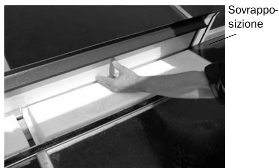
Fig. 108: Applicare le lamiere intermedie
