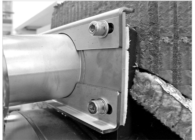
Fig. 2: Reinforcing the exhaust connection flange
