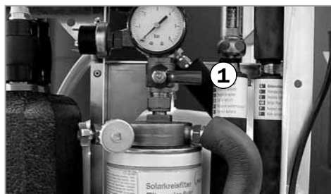
Ball valve over the solar filter closed
