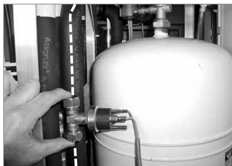
Determining the installation position of the pressure switch on the solar return
