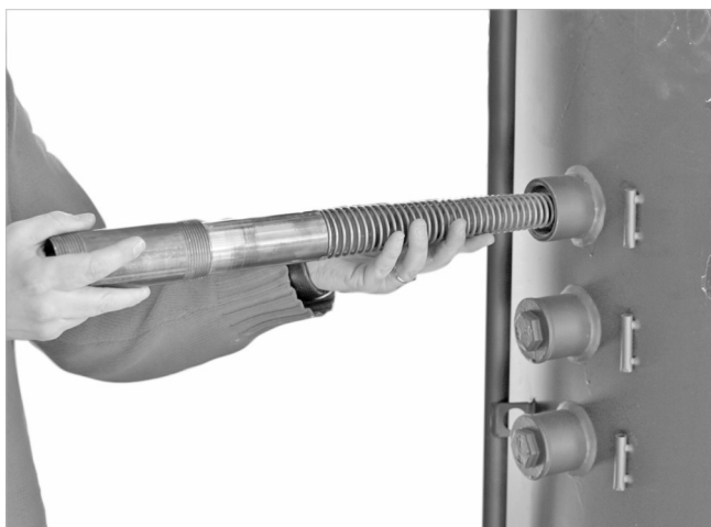
Fig. 3: Inserting and sealing the charging lance
