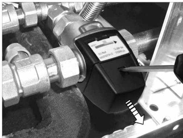
Fig. 6: Removing the cap from the TMV
