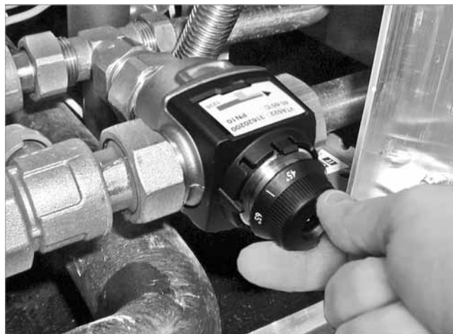
Fig. 7: Setting the TMV
