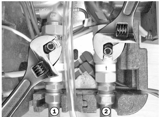
Fig. 8: Ball valves half-open/fully open
