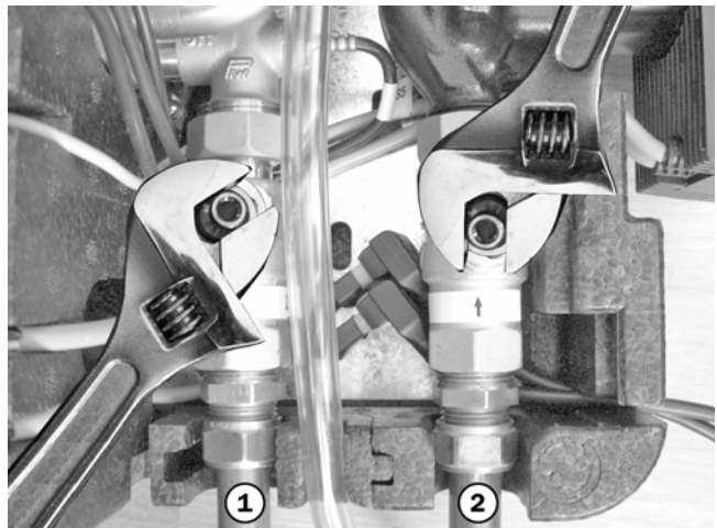
Fig. 8: Ball valves half-open/fully open
