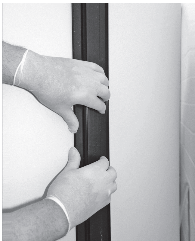
Fig. 8: Close the insulation sections
