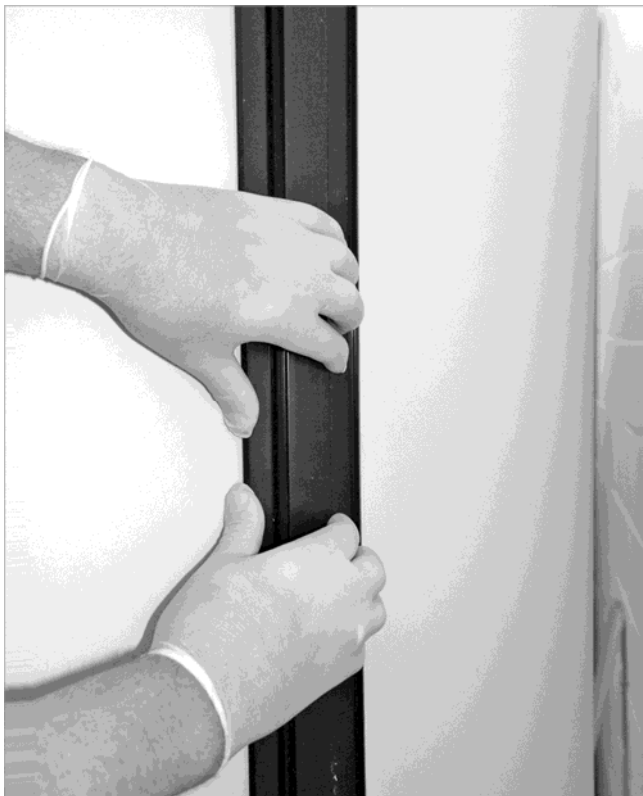
Fig. 8: Close the insulation sections
