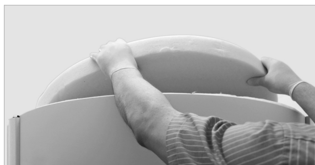
Fig. 9: Colocar as tampas redondas
