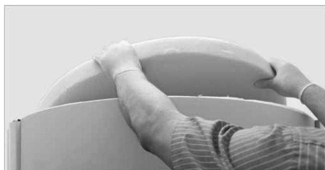
Fig. 9: Colocar as tampas redondas
