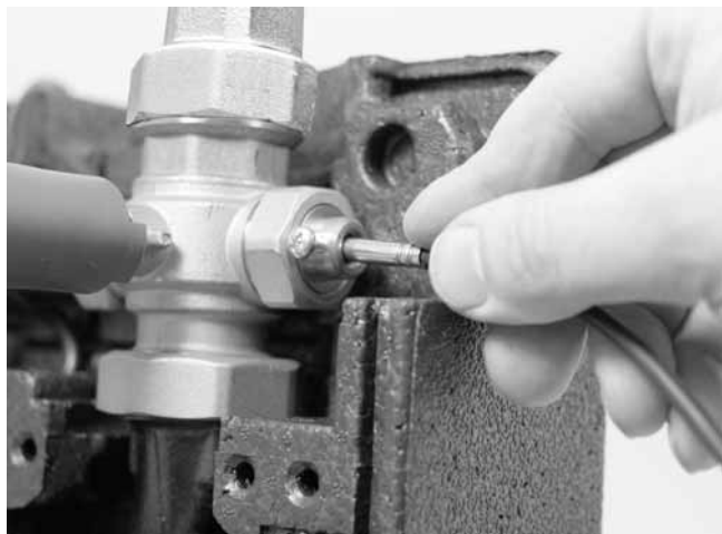
Fig. 43: Installing the flow temperature sensor
