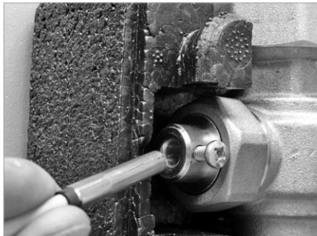
Fig. 3: Installing the return temperature sensor
