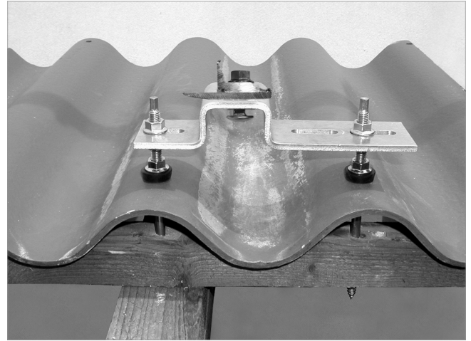
Fig. 19: Installed roof-mount frame (Method B)
