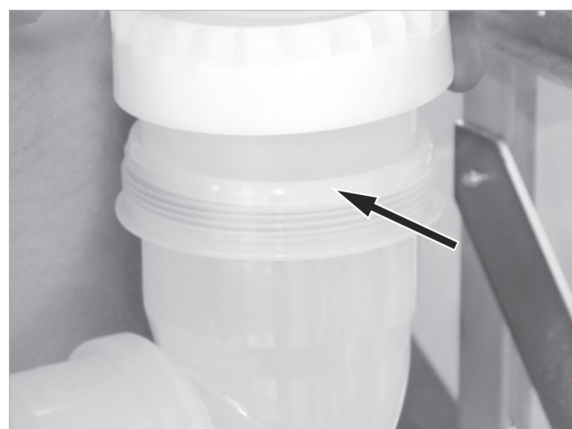
Fig. 15: Screwing on the straightly aligned exhaust elbow
