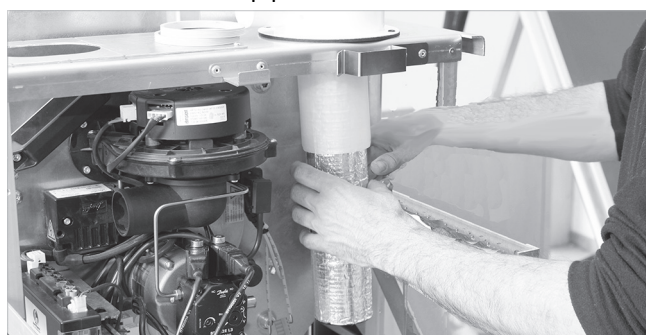
Fig. 11: Inserting the internal pipe silencer
