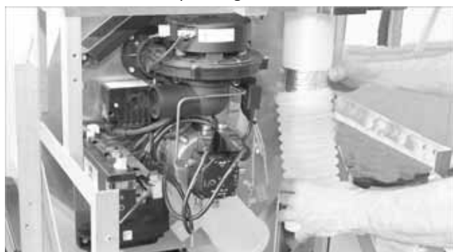
Fig. 12: Connecting the exhaust connection piece
