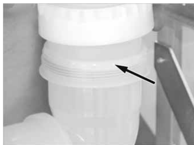
Fig. 15: Screwing on the straightly aligned exhaust elbow
