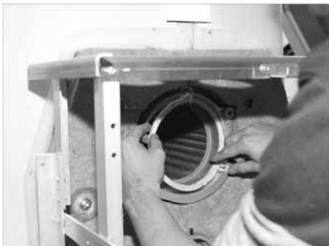
Fig. 1: Inserting the burner sealing cable
