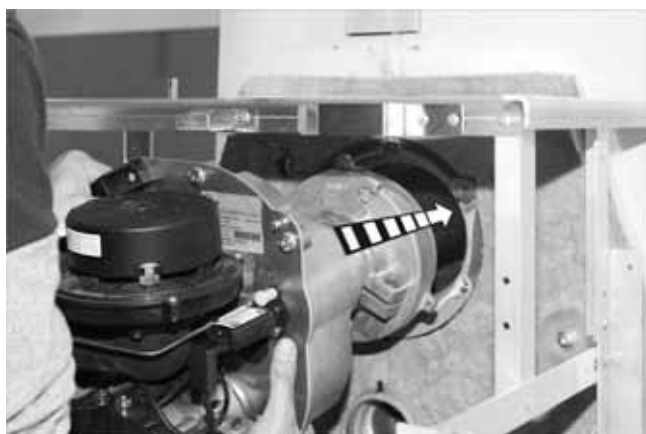
Fig. 7: Fitting the burner
