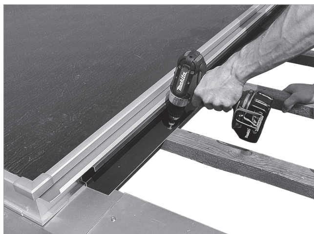
Fig. 52: Pushing the connecting plate down until it locks into the place and screwing it onto the battens
