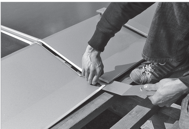
Fig. 80: Pushing the lower plate of the connector under the top flashing
