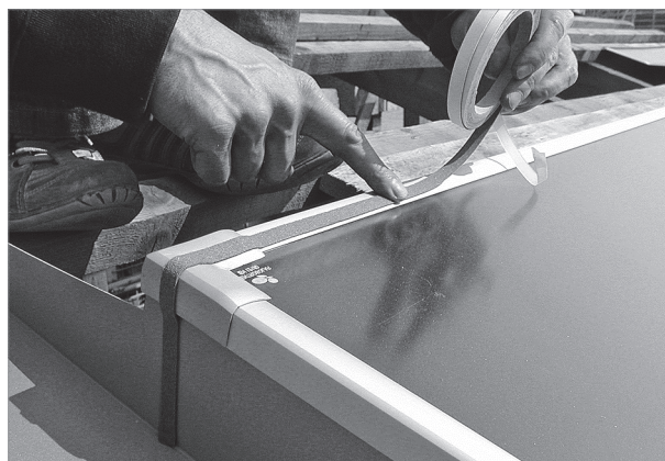
Fig. 68: Sticking joint sealing strip on the upper edge along the entire width
