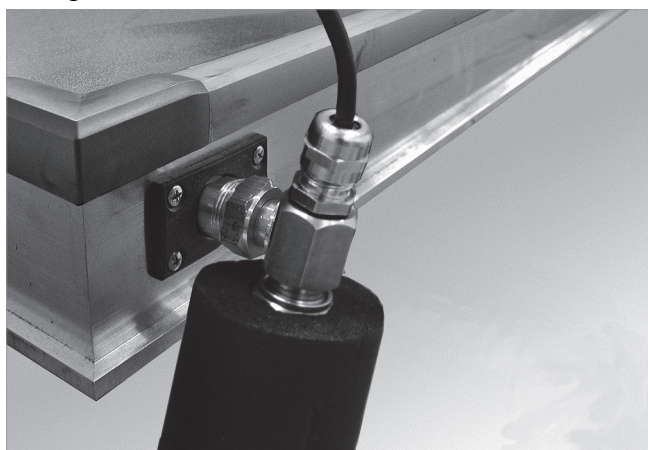
Fig. 91: Install sensor (solar flow)
