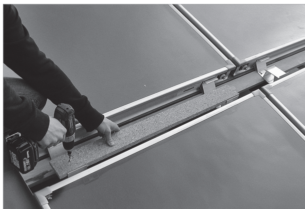
Fig. 67: Screwing intermediate flashing supports onto collector spacers
