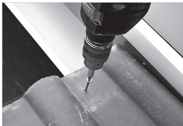
Fig. 87: Fastening the tile next to the side flashing
