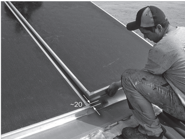
Fig. 53: Setting down the next collector and pushing it down against the retaining plate
