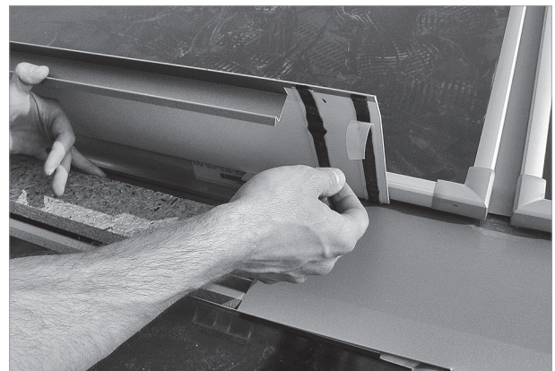
Fig. 74: Installing additional plates: removing the protective strips before positioning
