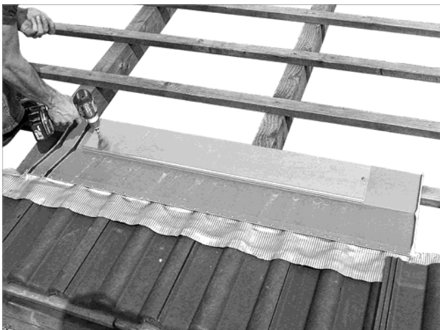
Fig. 46: Positioning the first plate on the right and screwing it on
