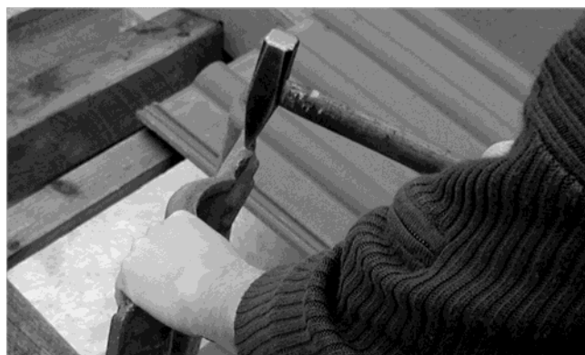
Fig. 86: Removing stoppers as necessary
