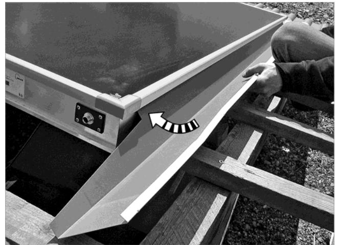
Fig. 55: Positioning the flashing next to the slot under the clip profile, then attaching it to the collector
