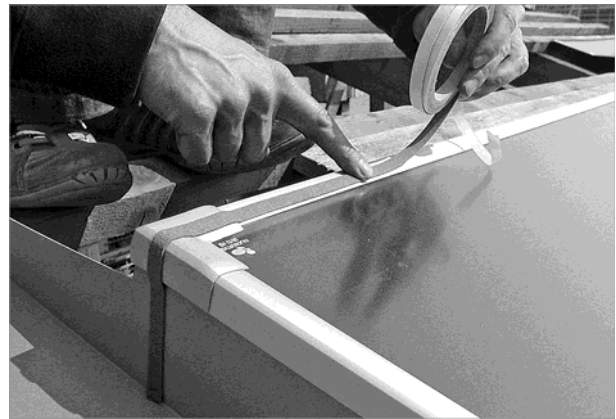
Fig. 68: Sticking joint sealing strip on the upper edge along the entire width
