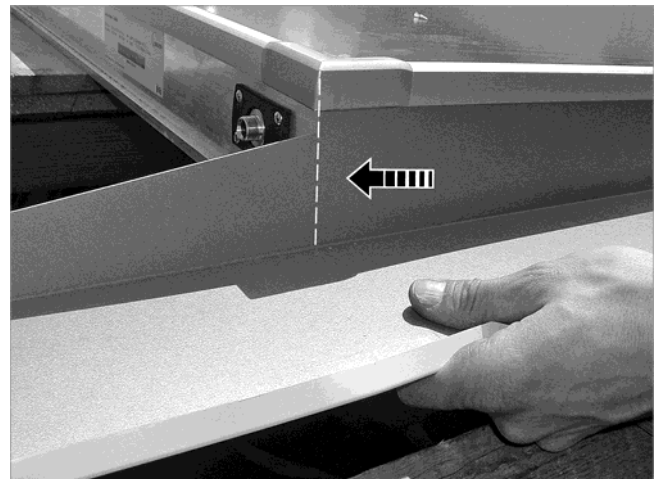
Fig. 56: Sliding the upper part of the side flashing up until it reaches the stop
