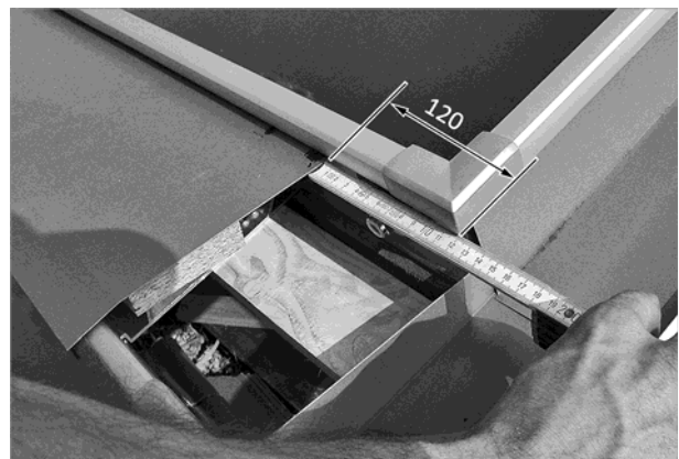
Fig. 70: Positioning the plate at the correct distance from the outer edge
