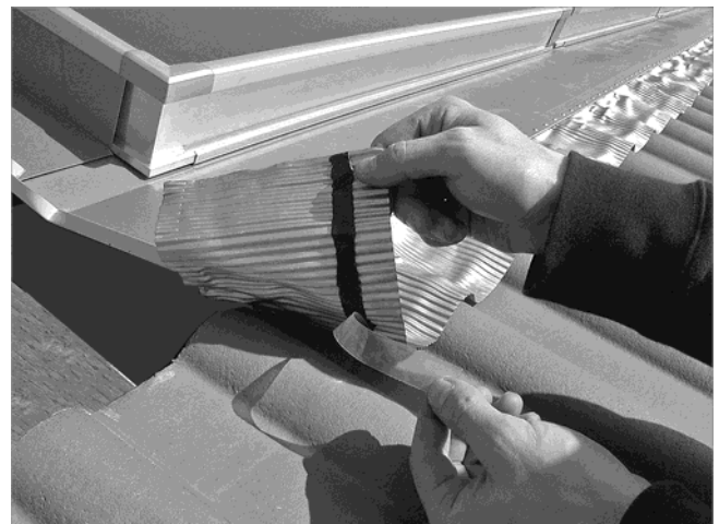
Fig. 48: Removing the protective strips and pressing on the lead aprons
