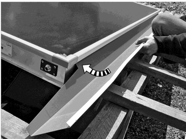
Fig. 63: Positioning the flashing next to the slot under the clip profile, then attaching it to the collector
