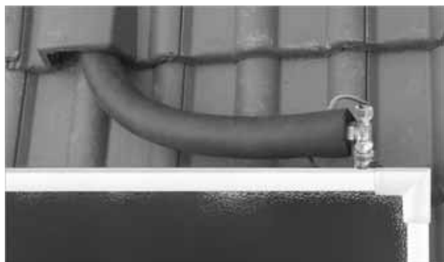
Fig. 93: Connect flow
