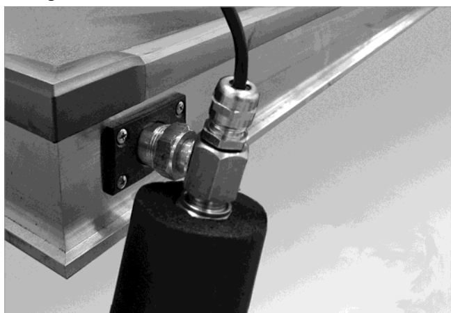
Fig. 91: Install sensor (solar flow)
