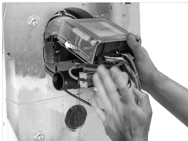
Fig. 8: Fitting the burner
