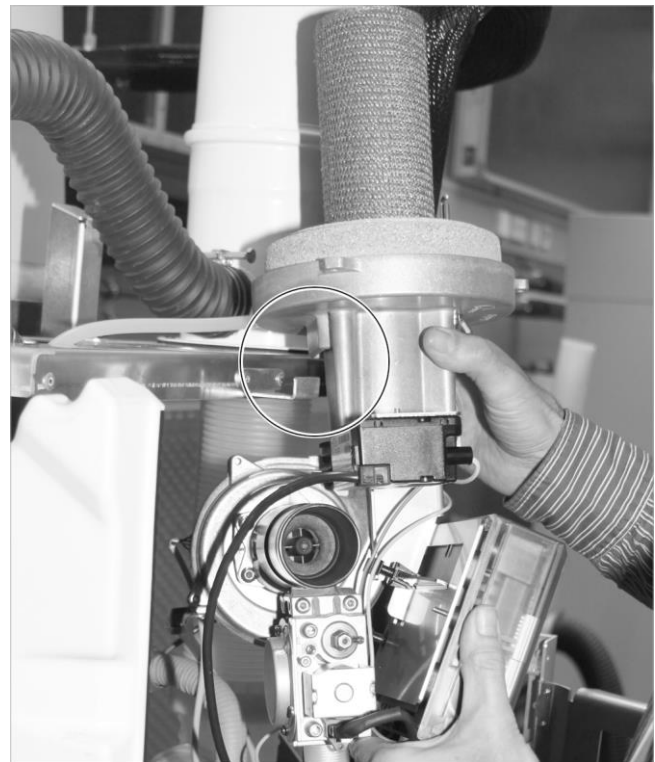
Fig. 31: Burner in maintenance position on the console
