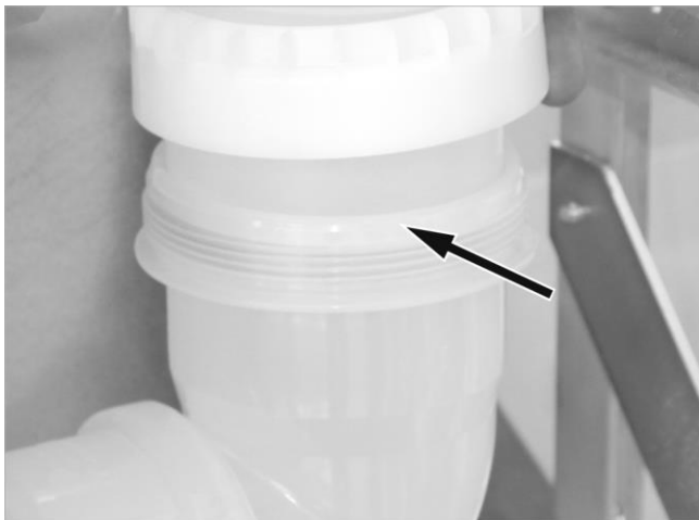
Fig. 19: Screwing on the straightly aligned exhaust elbow
