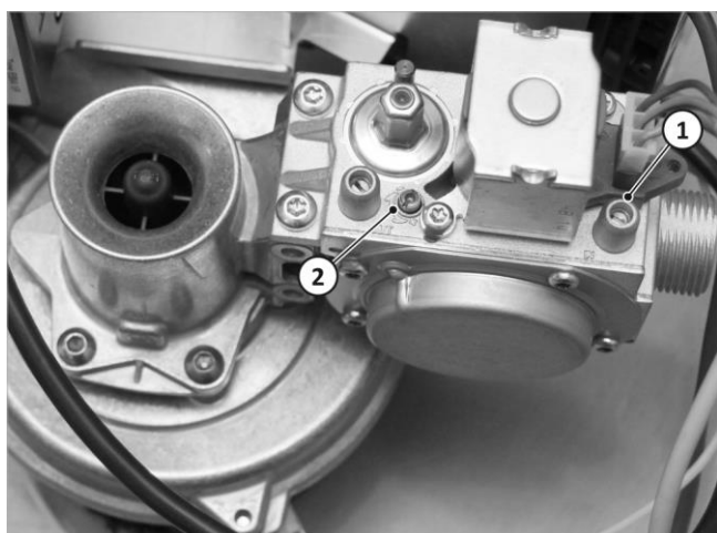
Fig. 30: Setting the burner
