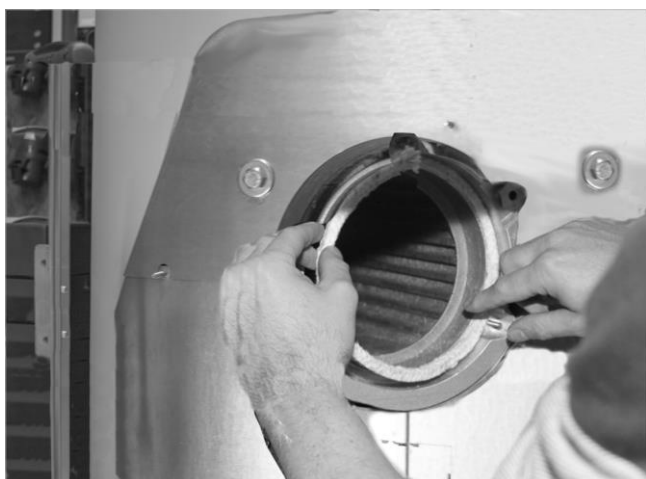
Fig. 6: Inserting the burner sealing cable (push up)
