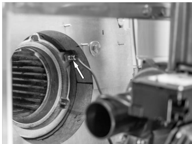
Fig. 7: Inserting the eSTB
