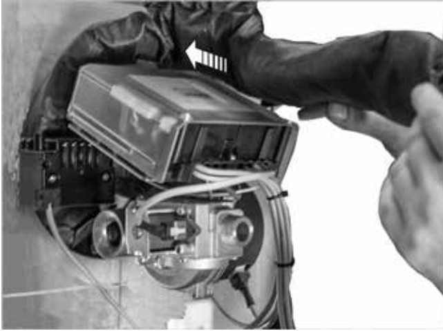
Fig. 9: Filling the recess on the burner flange
