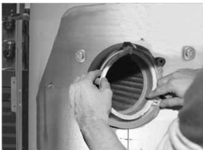
Fig. 6: Inserting the burner sealing cable (push up)
