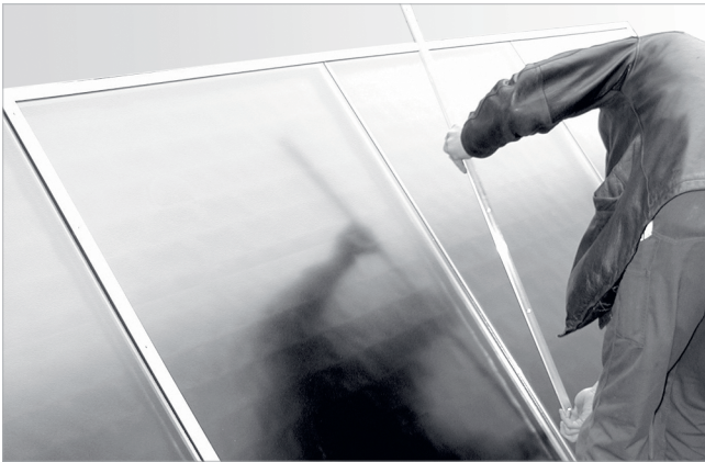
Fig. 37: Installing crossmember cover strips
