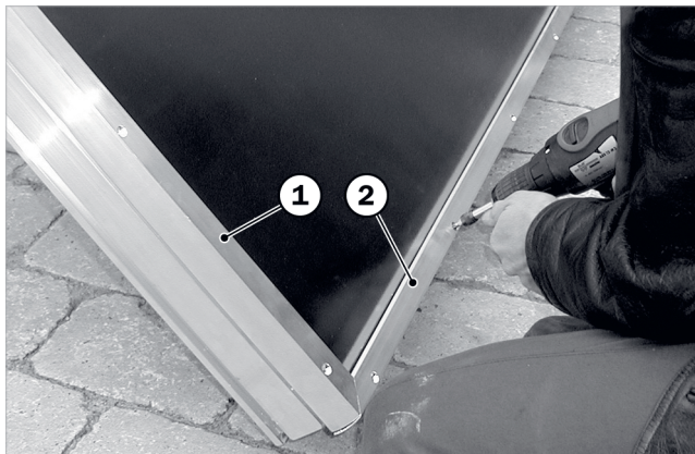
Fig. 34: Positioning, aligning and screwing on clip profiles
