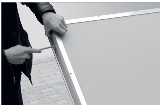
Fig. 32: Removing the clip profiles and cardboard covers
