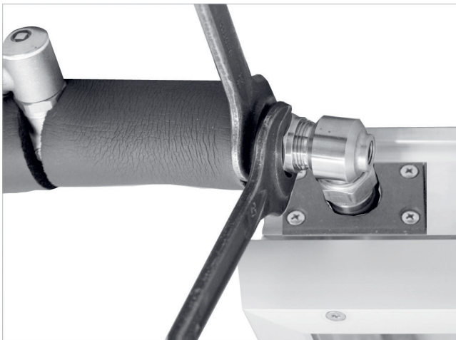
Fig. 57: Top connection: Solar flow
