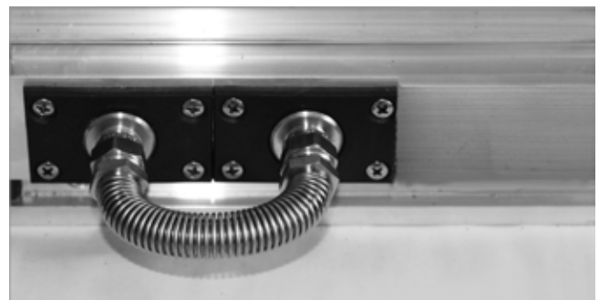
Fig. 45: Installed connection elbow
