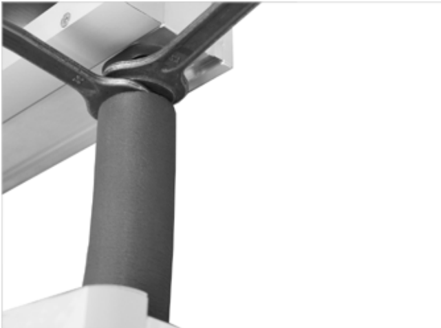
Fig. 60: Screwing VB-F-S-D-UE to the upper connection
