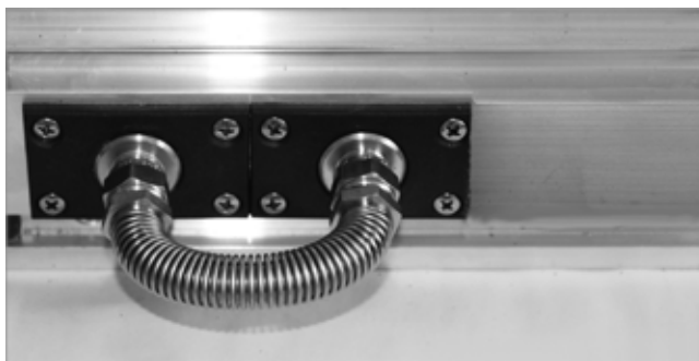
Fig. 54: Installed connection elbow
