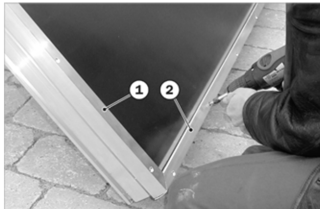
Fig. 34: Positioning, aligning and screwing on clip profiles
