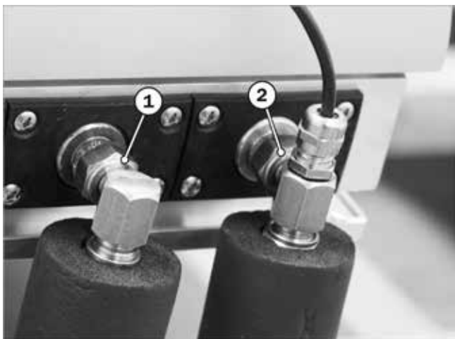
Fig. 71: Fitted collector sensor, SolvisFera Integral
