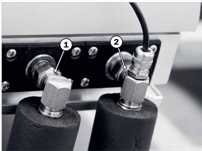
Fig. 71: Sensor sumergible montado, SolvisFera Integral
