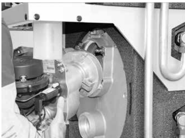
Fig. 70: Fitting the burner
