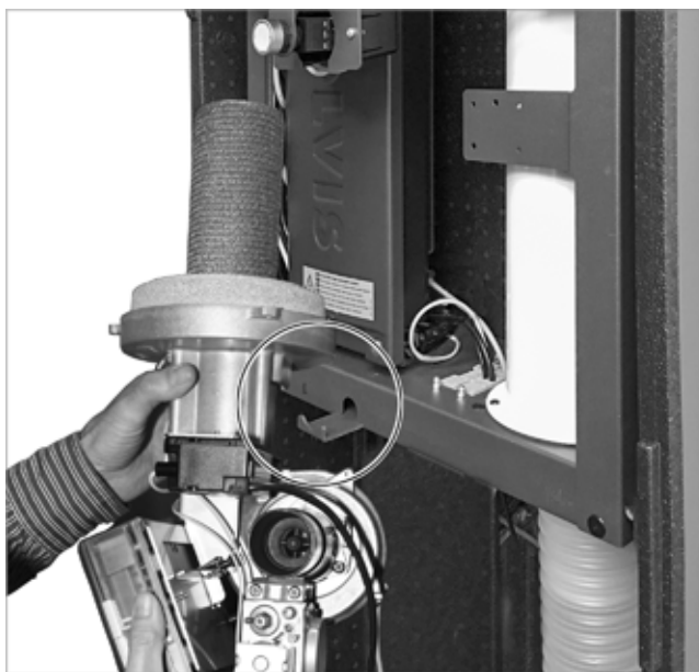
Fig. 141: Attaching the burner to the console (maintenance position)
