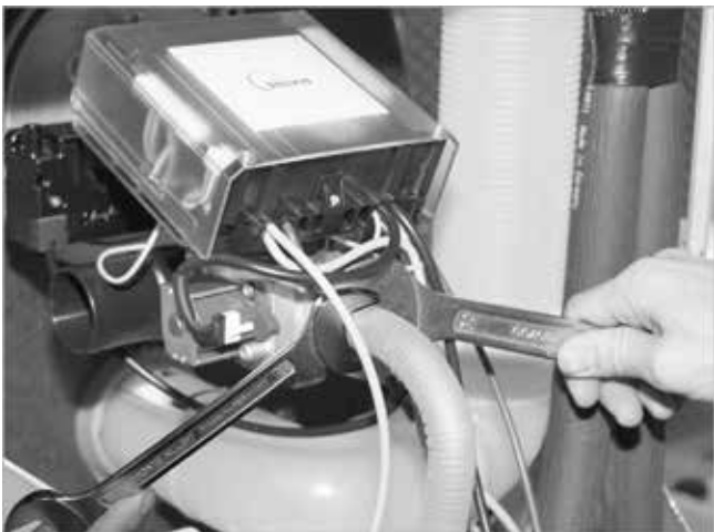
Fig. 60: Connecting the gas line
