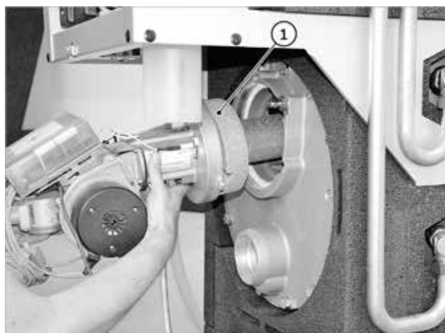
Fig. 49: Fitting the burner
