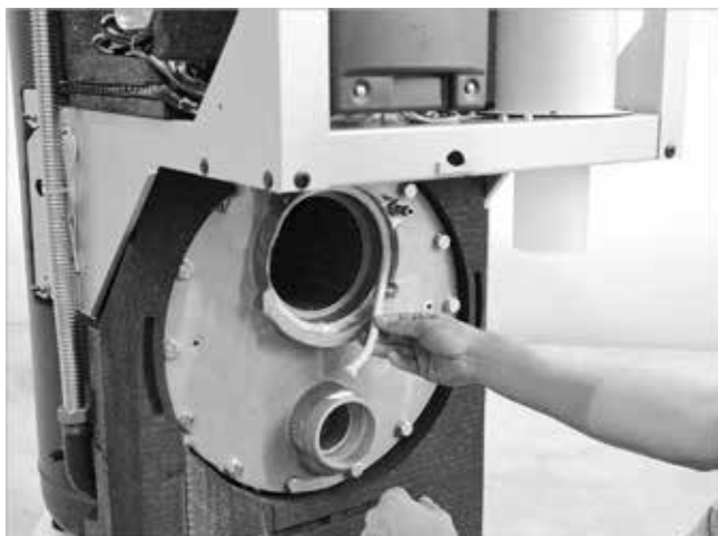
Fig. 46: Inserting the burner sealing cable
