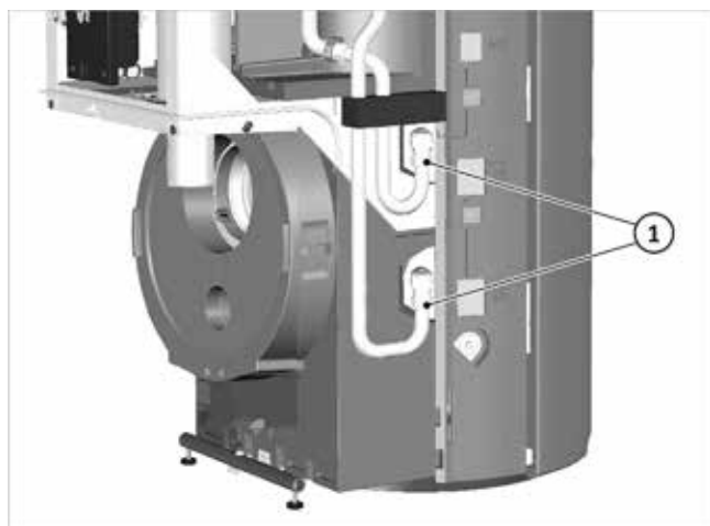
Fig. 31: Checking/retightening the heating circuit station connections
