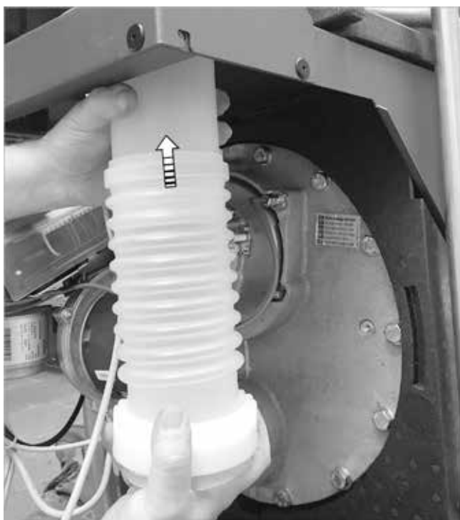
Fig. 88: Connecting the exhaust connection piece onto the flue duct
