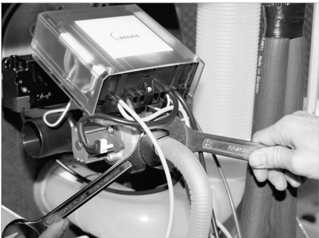
Fig. 60: Connecting the gas line
