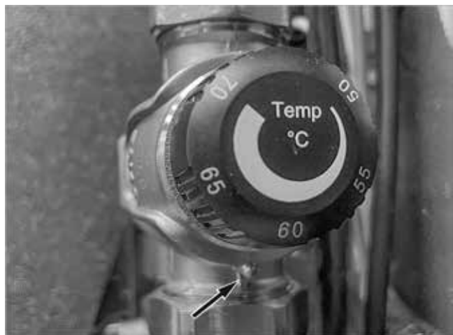
Fig. 60: Setting the TMV
