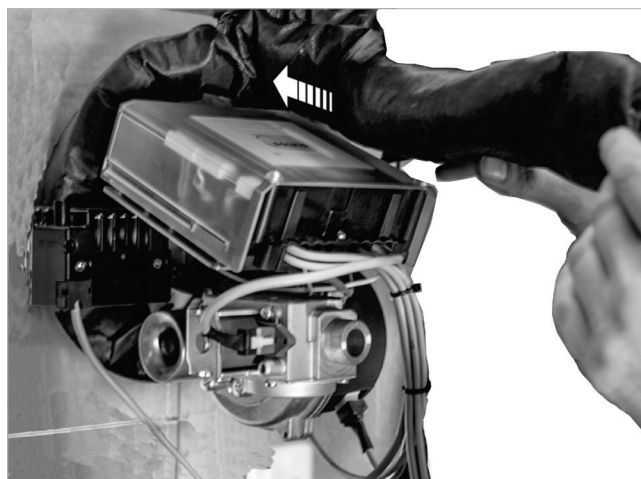
Fig. 29: Filling the recess on the burner flange
