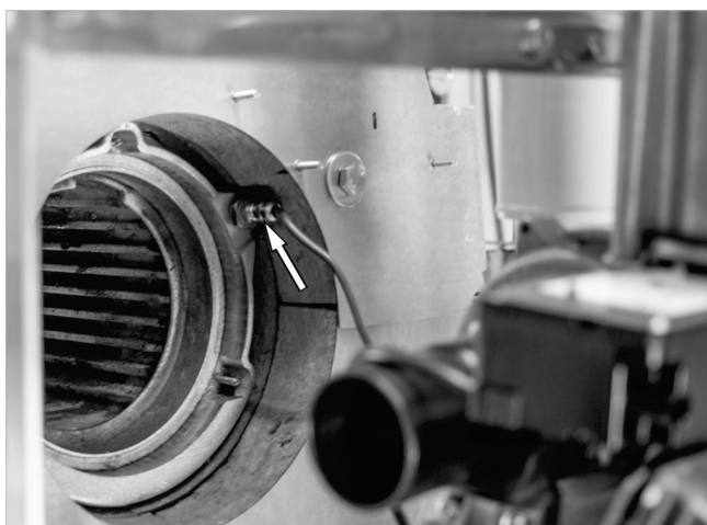
Fig. 27: Inserting the eSTB
