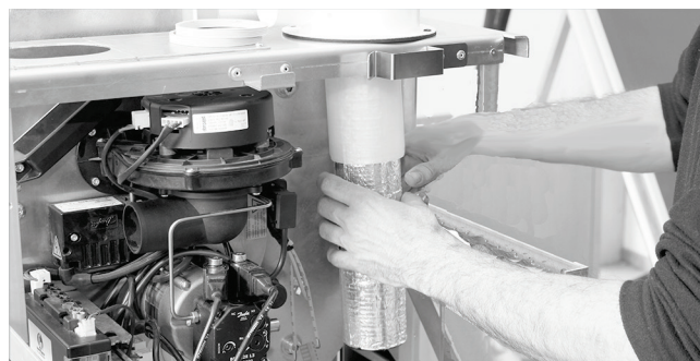
Fig.59: Inserting the internal pipe silencer
