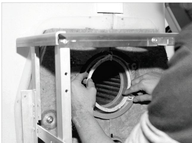
Fig. 49: Inserting the burner sealing cable (push up)
