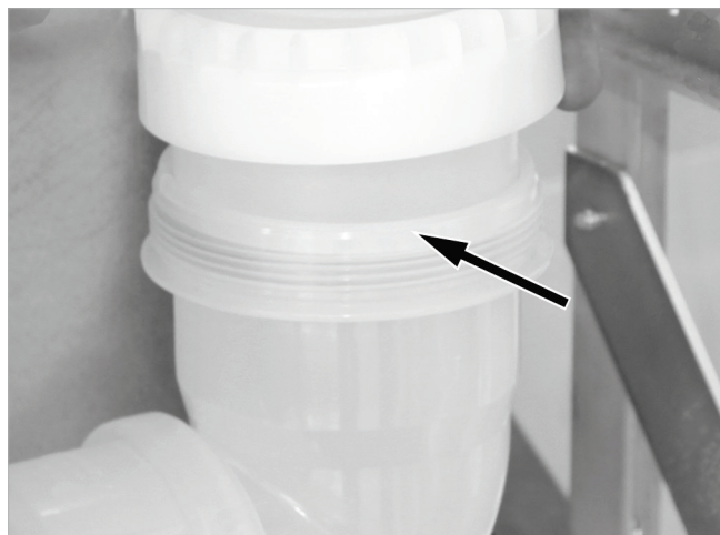
Fig. 63: Screwing on the straightly aligned exhaust elbow
