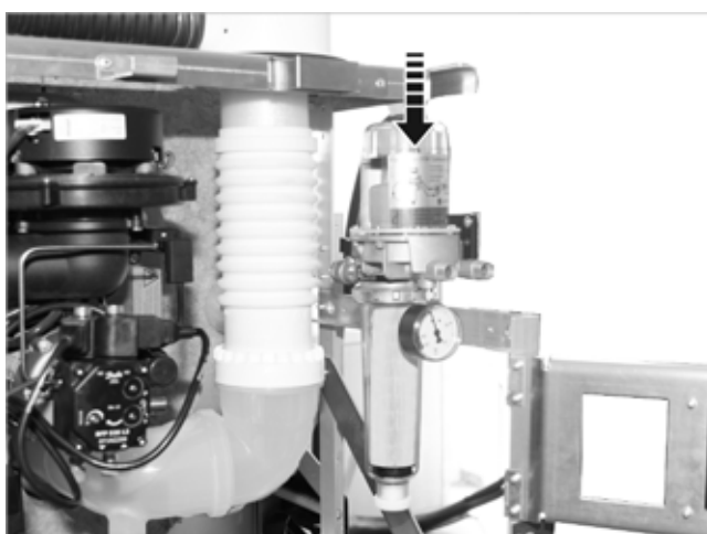
Fig. 65: Oil filter fitted
