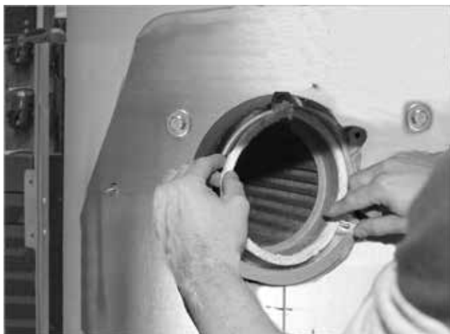
Fig. 26: Inserting the burner sealing cable (push up)
