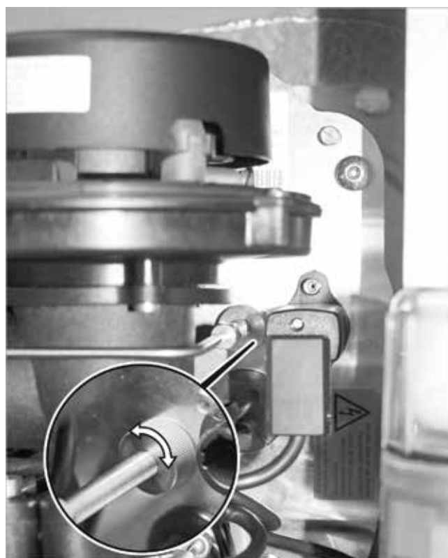
Fig. 120: Knurled nut (limit stop for oil pipe/nozzle fitting)
