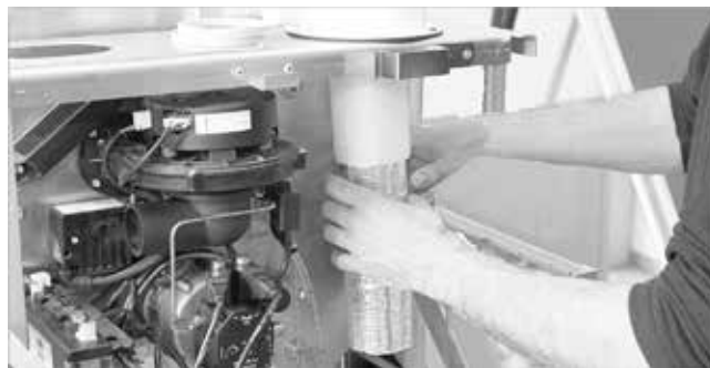
Fig.59: Inserting the internal pipe silencer
