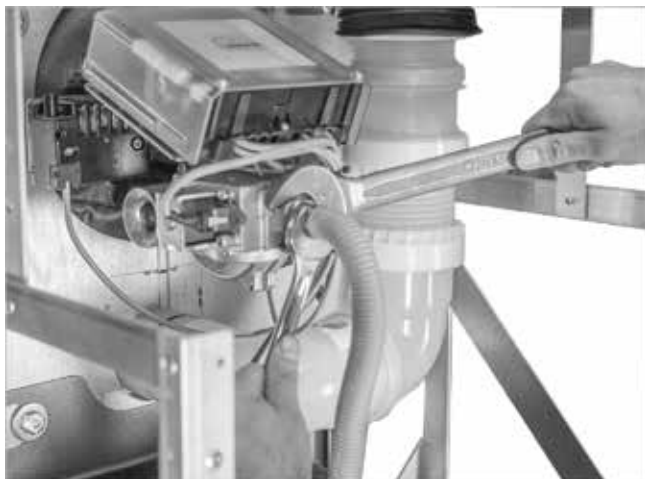
Fig. 43: Connecting the gas line
