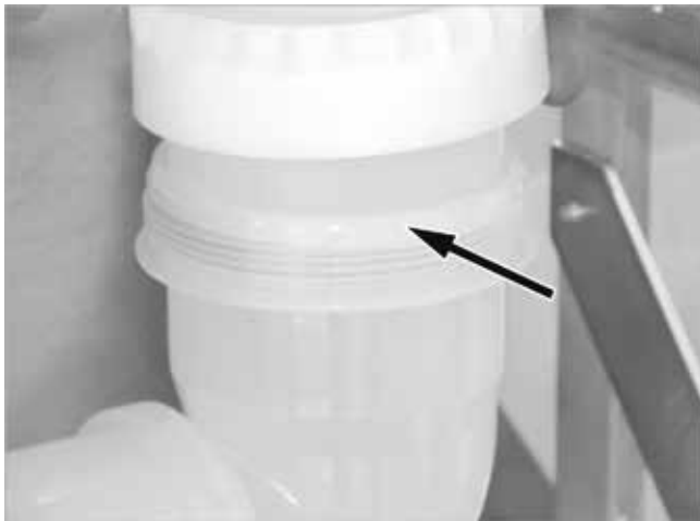
Fig. 39: Screwing on the straightly aligned exhaust elbow
