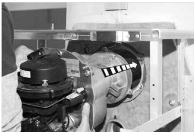
Fig. 55: Fitting the burner
