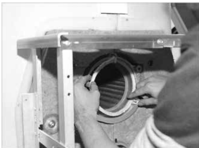
Fig. 49: Inserting the burner sealing cable (push up)
