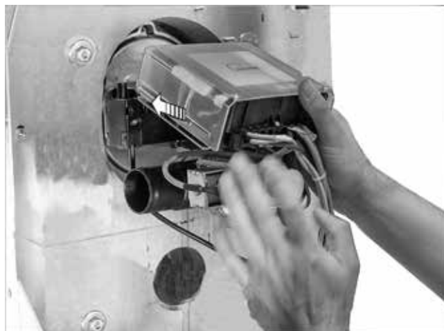
Fig. 28: Fitting the burner
