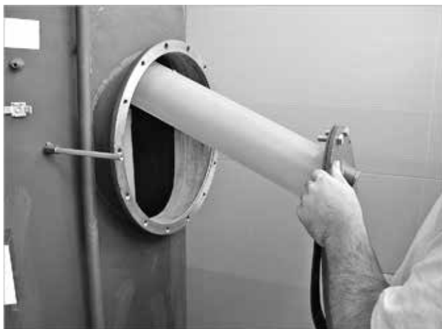
Fig. 3: Inserting the flange cover
