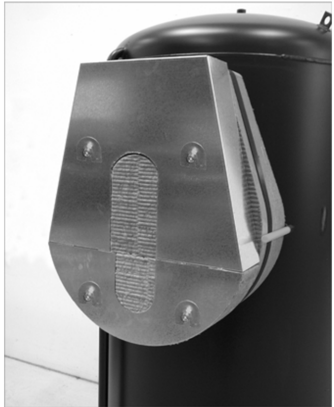
Fig. 1: Removing the flange insulation
