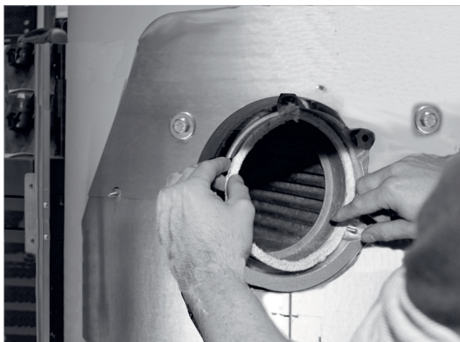
Fig. 30: Inserting the burner sealing cable (push up)
