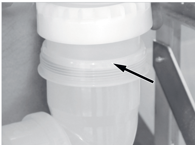
Fig. 66: Screwing on the straightly aligned exhaust elbow
