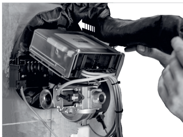
Fig. 33: Filling the recess on the burner flange
