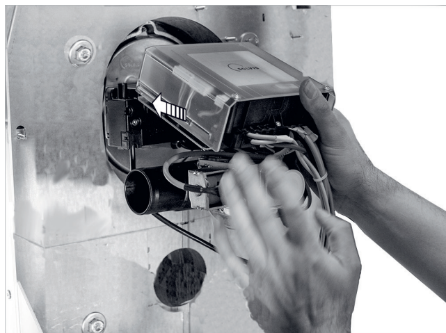
Fig. 32: Fitting the burner
