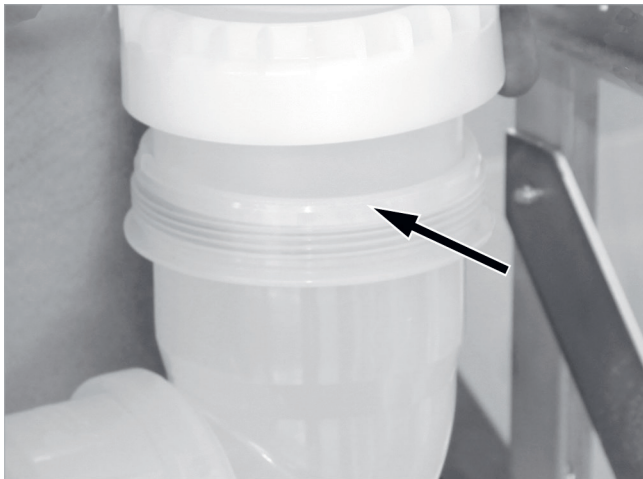
Fig. 43: Screwing on the straightly aligned exhaust elbow
