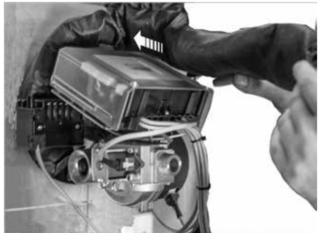
Fig. 33: Filling the recess on the burner flange
