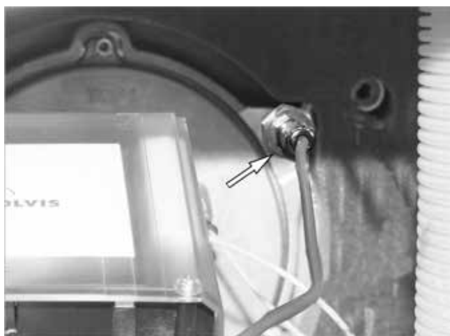
Fig. 115: Inserting the eSTL
