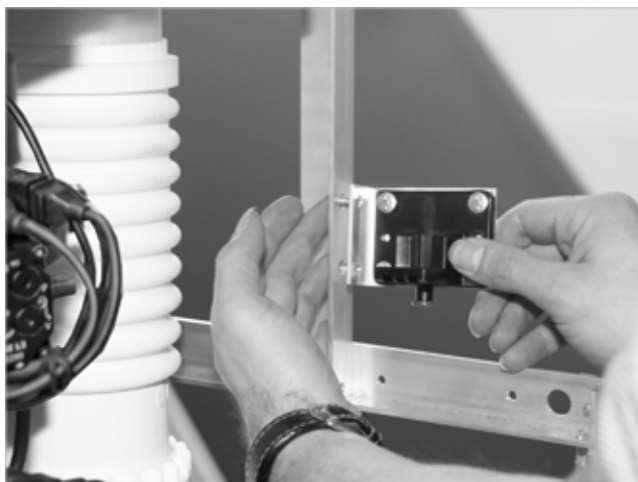
Fig. 67: Attaching the oil filter bracket
