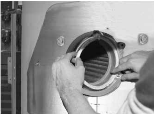
Fig. 30: Inserting the burner sealing cable (push up)
