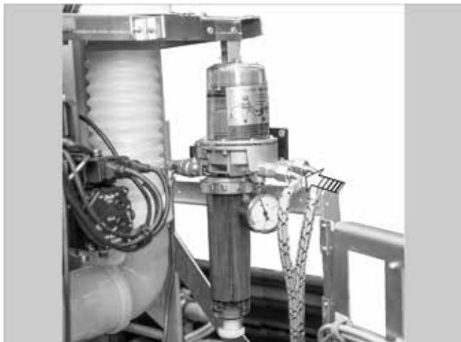
Fig. 69: Connecting the oil pipes
