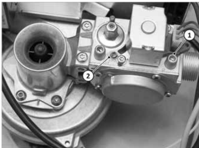
Fig. 103: Setting the burner
