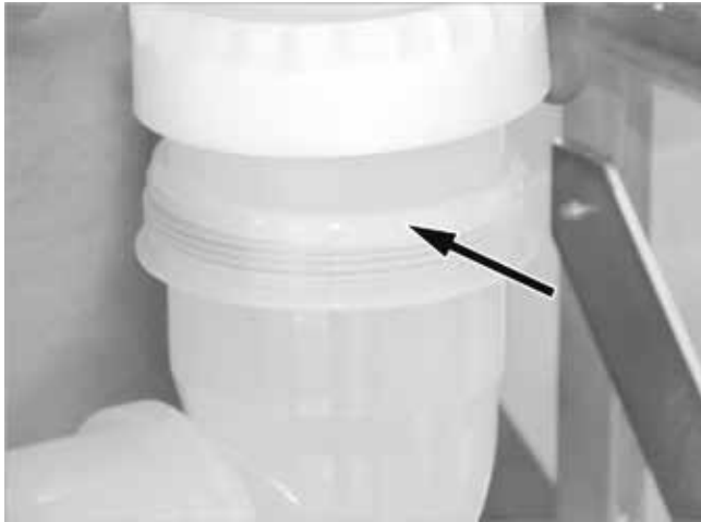
Fig. 43: Screwing on the straightly aligned exhaust elbow
