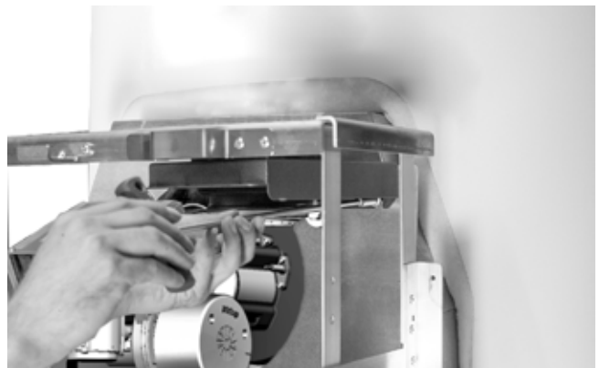
Fig. 38: Screwing the bellows seal bracket tightly
