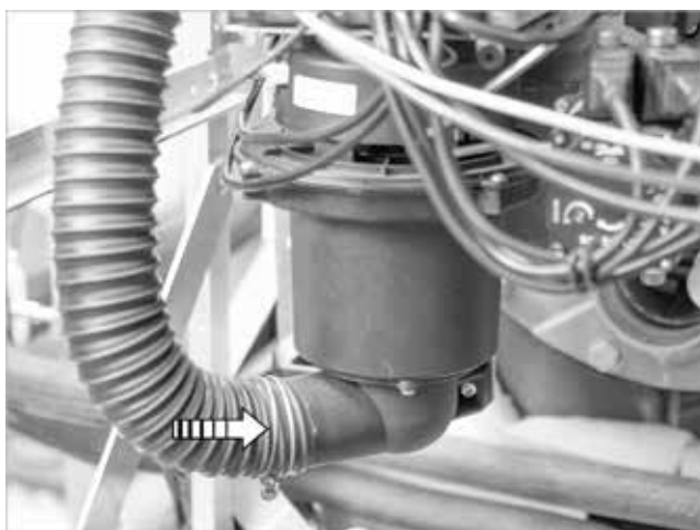
Fig. 59: Attaching the air supply hose to the blower
