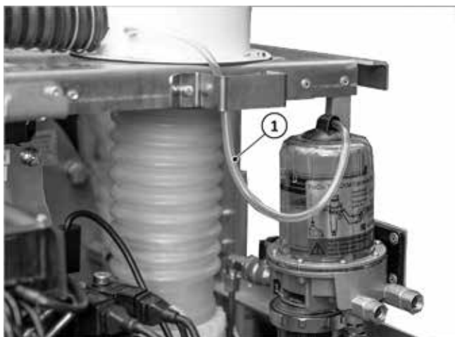
Fig. 71: Bleeder tube installed
