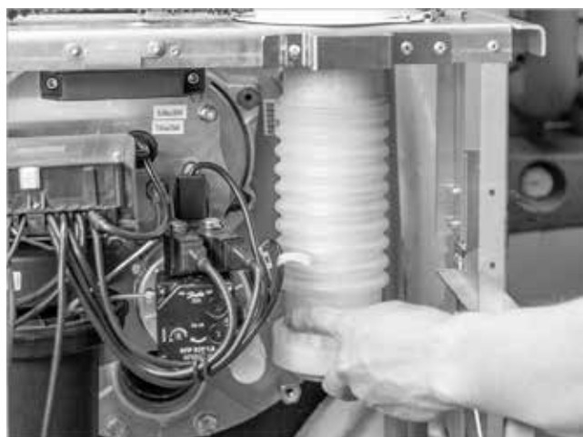
Fig. 64: Aligning the exhaust connection pipe section
