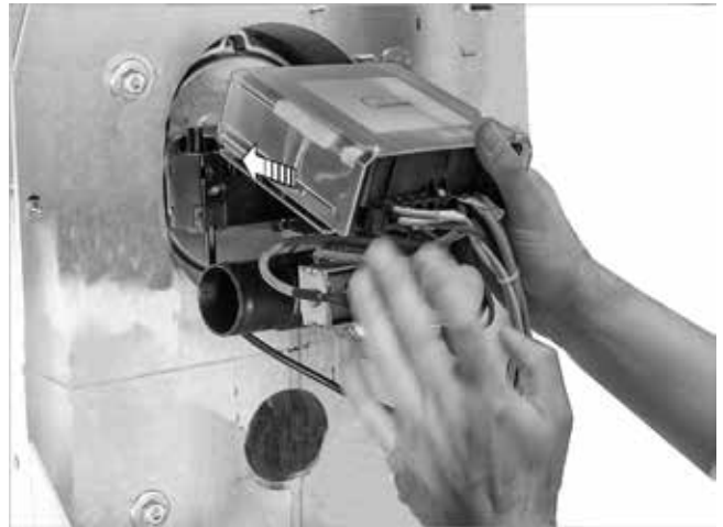
Fig. 32: Fitting the burner
