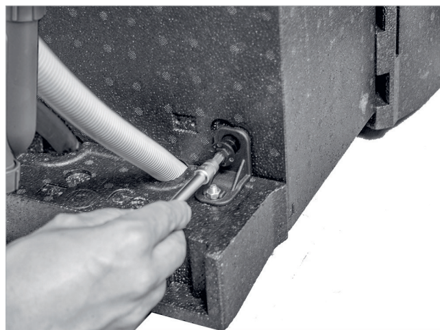
Fig. 92: Fastening the bracket
