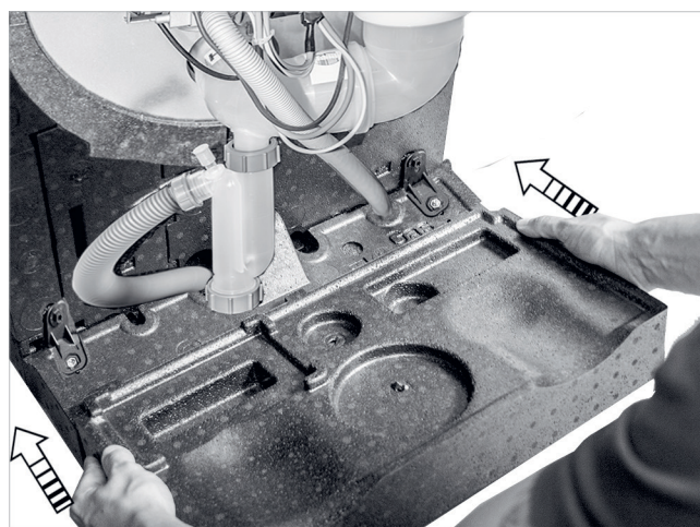
Fig. 93: Connecting the front base section
