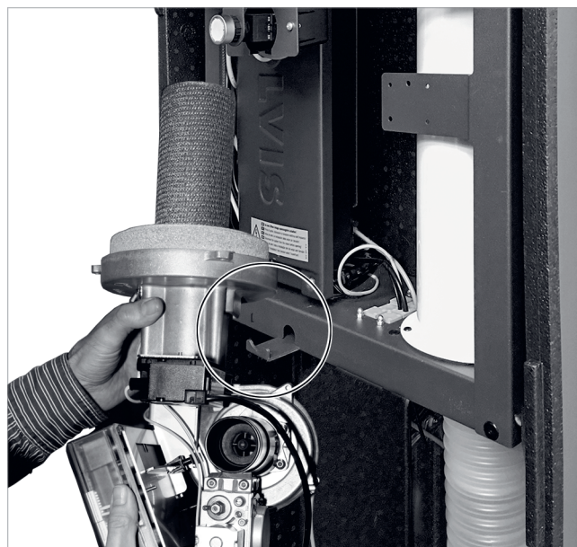
Fig. 136: Attaching the burner to the console (maintenance position)
