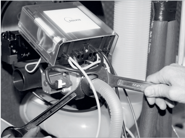
Fig. 60: Connecting the gas line
