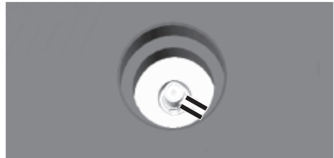
Fig. 135: Bleeder hose on the bleeder
