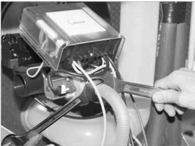
Fig. 60: Connecting the gas line
