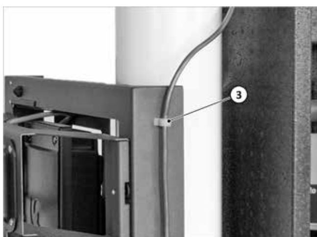
Fig. 79: Fastening the oil supply line to the frame
