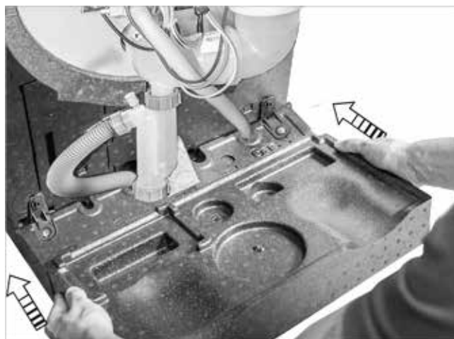
Fig. 93: Connecting the front base section
