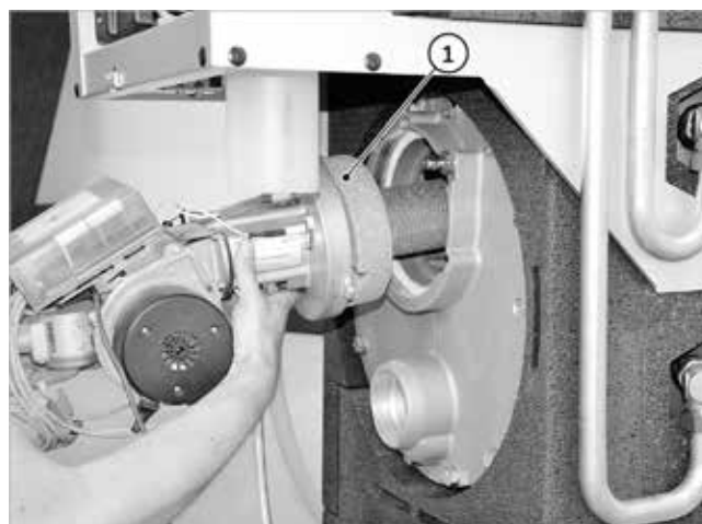
Fig. 49: Fitting the burner
