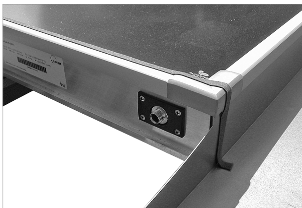
Fig. 79: Sticking the joint sealing strip on the upper edge along the entire width of the profile
