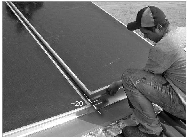
Fig. 54: Setting down the next collector and pushing it down against the retaining plate
