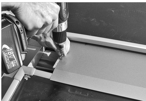
Fig. 72: Screwing on the intermediate flashing at least 10 mm from the outer left edge
