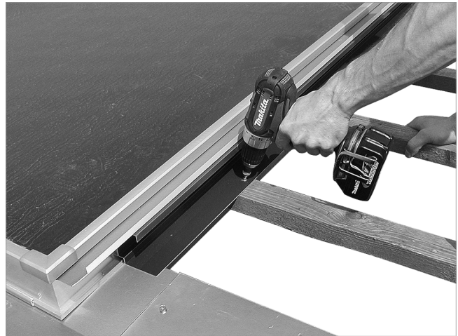
Fig. 53: Pushing the connecting plate down until it locks into the place and screwing it onto the battens
