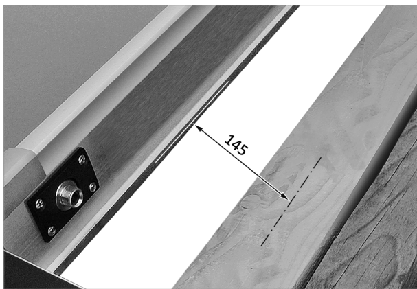
Fig. 60: For additional rows of collectors, install additional sheeting above the collector if necessary.
