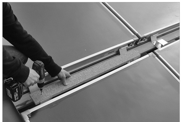
Fig. 68: Screwing intermediate flashing supports onto collector spacers
