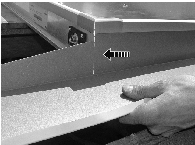
Fig. 57: Sliding the upper part of the side flashing up until it reaches the stop
