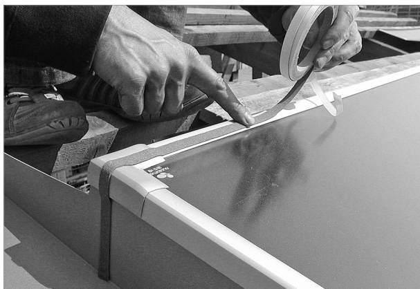
Fig. 69: Sticking joint sealing strip on the upper edge along the entire width
