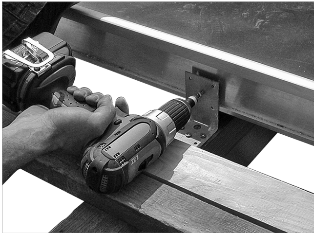
Fig. 51: Fastening the collector to the rafter on the front at the top
