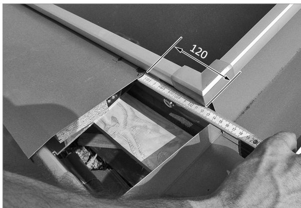
Fig. 71: Positioning the plate at the correct distance from the outer edge
