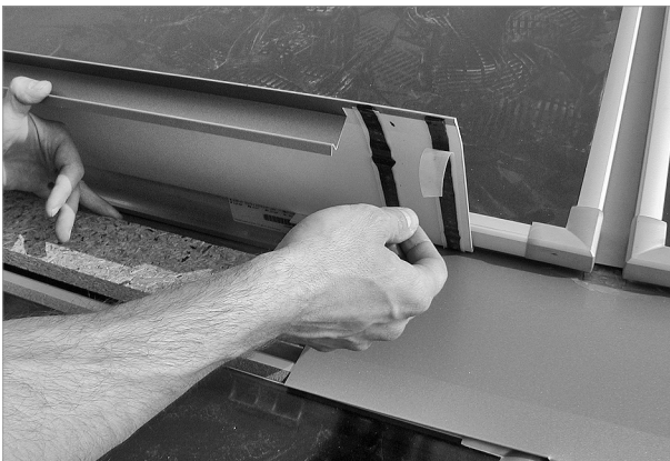
Fig. 75: Installing additional plates: removing the protective strips before positioning
