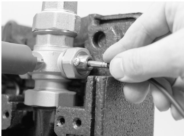
Fig. 44: Installing the flow temperature sensor
