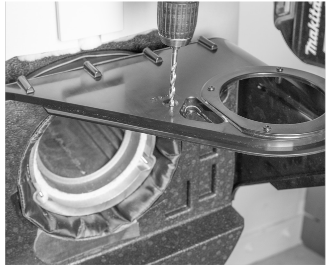
Fig. 52: 5.2 mm hole diameter
