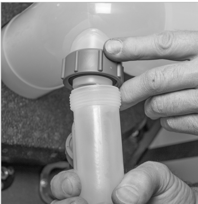
Fig. 86: Screw on condensate siphon hand-tight
