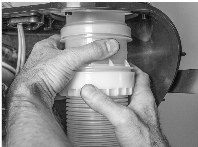
Fig. 82: Screw the flexible pipe to the flue pipe coupling
