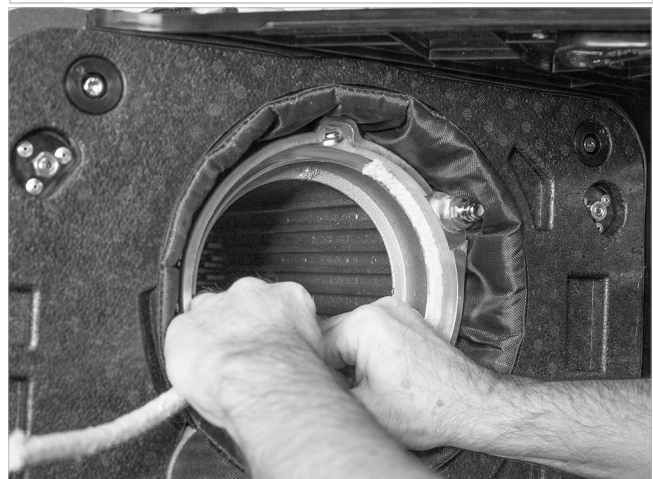
Fig. 38: Inserting the burner sealing cord, joint at 1 o'clock
