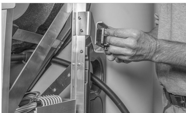
Fig. 64: Fix the mounting plate
