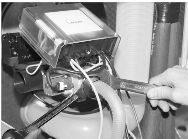
Fig. 45: Connecting the gas line
