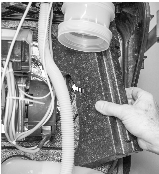
Fig. 92: Installing the right-hand front flange insulation (part II)
