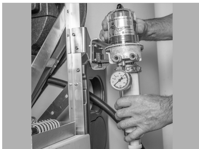
Fig. 65: Attaching the oil filter
