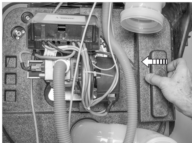
Fig. 93: Fitting the right-hand front flange insulation (part III)
