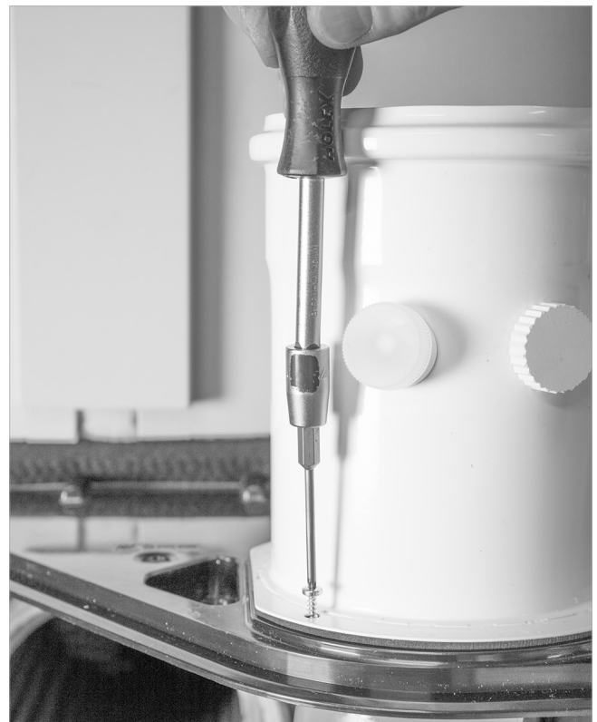
Fig. 53: Assembling the exhaust connection piece
