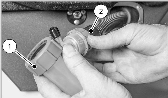
Fig. 84: Connecting the condensate siphon to the condensate hose
