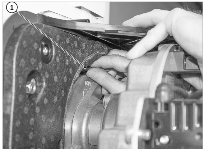
Fig. 61: Fix the burner with long nuts (1).
