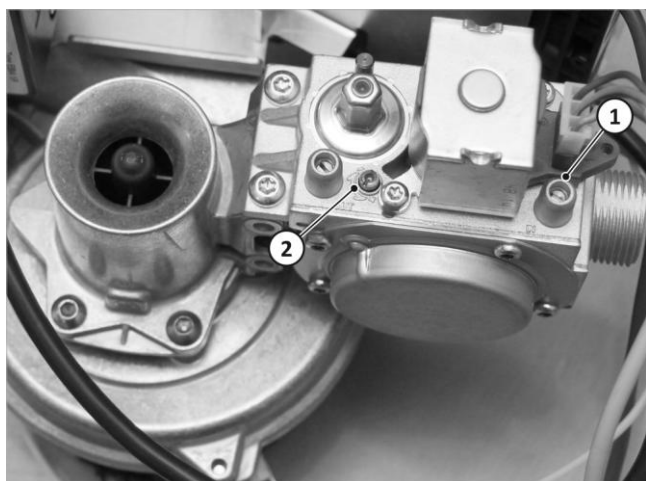
Fig. 119: Setting the burner
