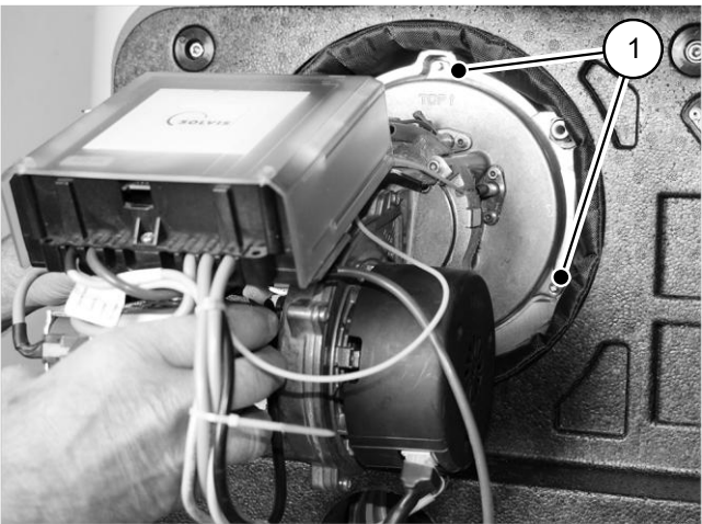
Fig. 52: Assemble the burner
