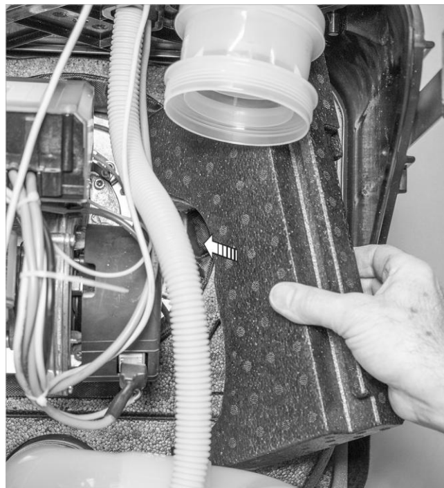
Fig. 98: Installing the right-hand front flange insulation (part II)
