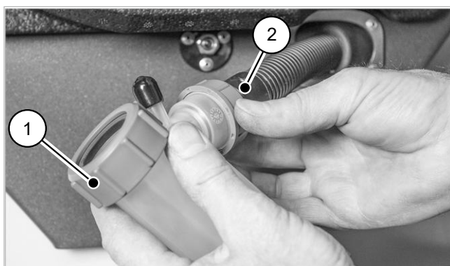
Fig. 86: Connecting the condensate siphon to the condensate hose
