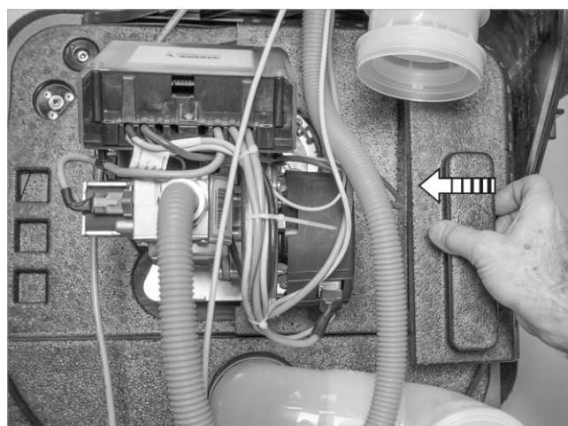
Fig. 99: Fitting the right-hand front flange insulation (part III)
