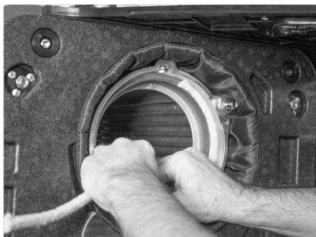
Fig. 48: Inserting the burner sealing cord, joint at 1 o'clock
