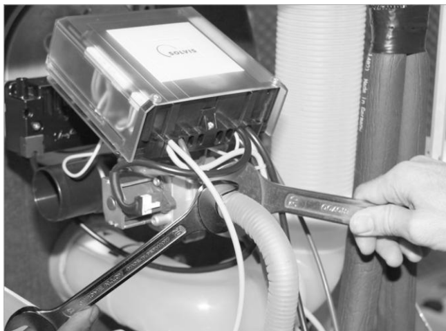
Fig. 55: Connecting the gas line
