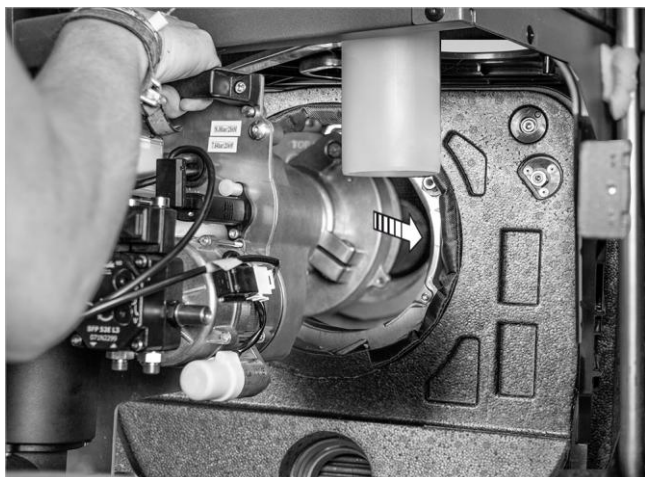
Fig. 65: Fitting the burner
