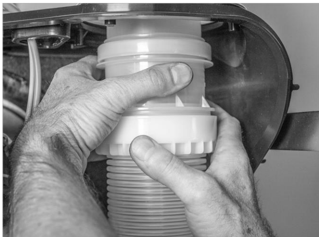
Fig. 85: Screw the flexible pipe to the flue pipe coupling
