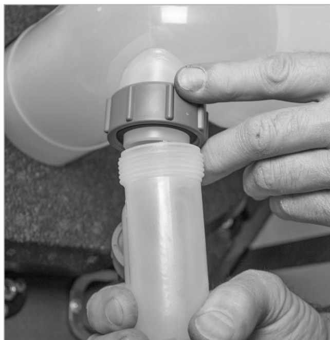
Fig. 88: Screw on condensate siphon hand-tight
