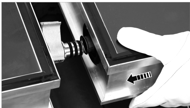
Fig. 43: Attaching collectors together
