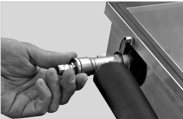
Fig. 49: Connecting solar flow
